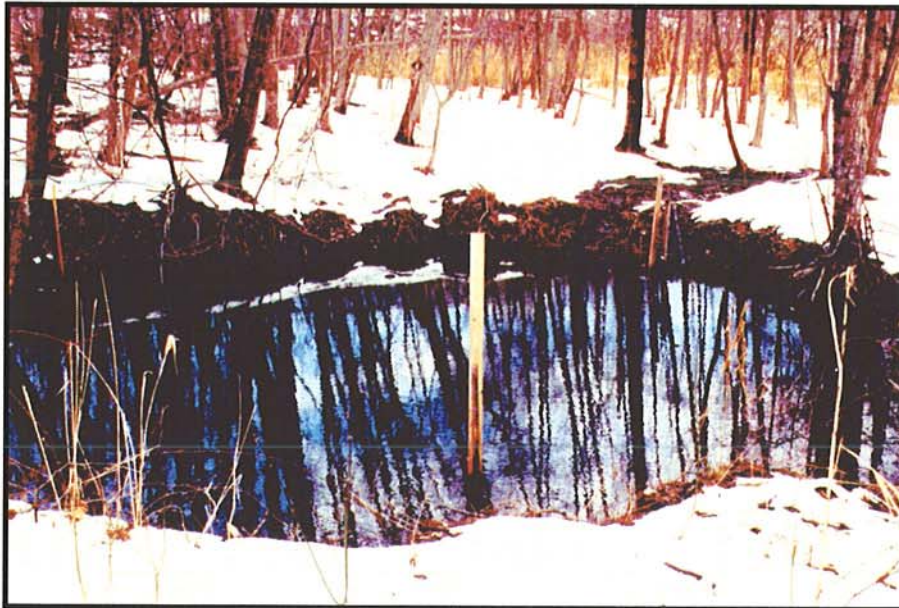
Six hundred feet above the fractured aqueduct, New York City drinking water fills this sinkhole in the forest floor near Roseton. Photo by William Wegner.
