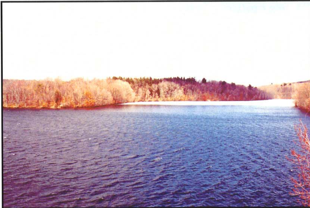
Westchester County's Kensico Reservoir - the terminal reservoir for 90% of New York City's drinking water supply. Photo by William Wegner.
