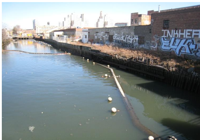
Figure 6: Boom in Gowanus Canal to catch floatable material
