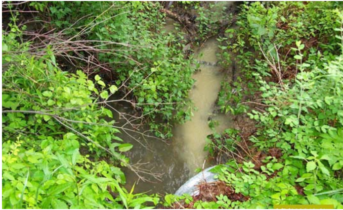
Muddy water from the construction of one single-family home enters the inlet of a neighbor’s pond in Southeast, New York.
