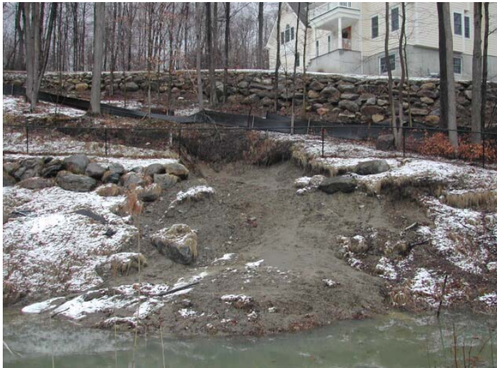
A sprawling subdivision in the Croton watershed. The developer has failed to maintain stormwater controls. Photo by William Wegner.
