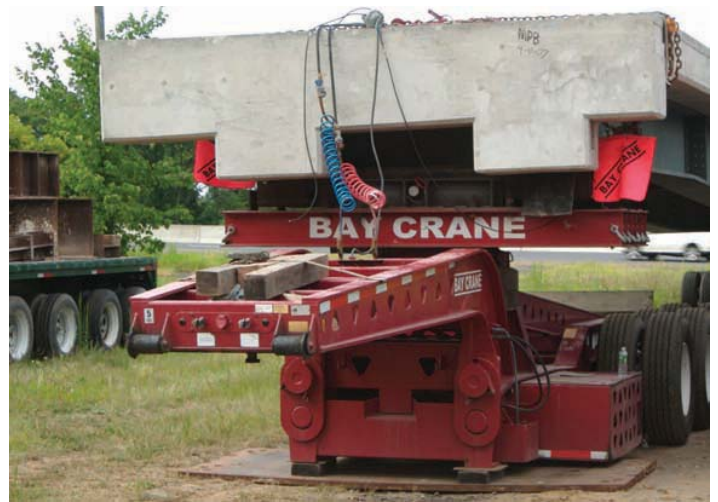
A $147 million deck replacement project began in September.
