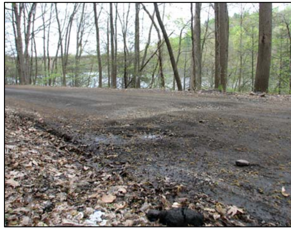
The Croton Dam Road runs adjacent to, and has the potential to send sediment into the City’s Croton Reservoir in the Town of Yorktown, Westchester County. Photo by Leila Goldmark.
