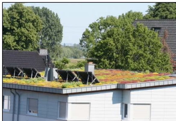
Green roofs are attractive and cost effective while also providing stormwater treatment.
