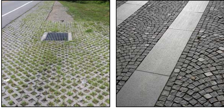
Biopavers (left) and other pervious pavers (right) allow stormwater to seep into the ground, helping to protect water quality and prevent flooding. Left photo by William Wegner.
