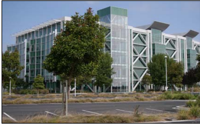
Vegetated filter strips (a type of bioretention) placed below grade easily capture and treat polluted runoff from parking lots while providing shade and enhancing the aesthetics of the space.
