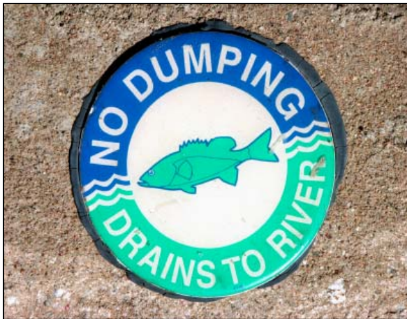
Marking storm drains effectively educates the public about where each drain discharges and also can help satisfy the MS4 permit requirements for pollution prevention/good housekeeping.
