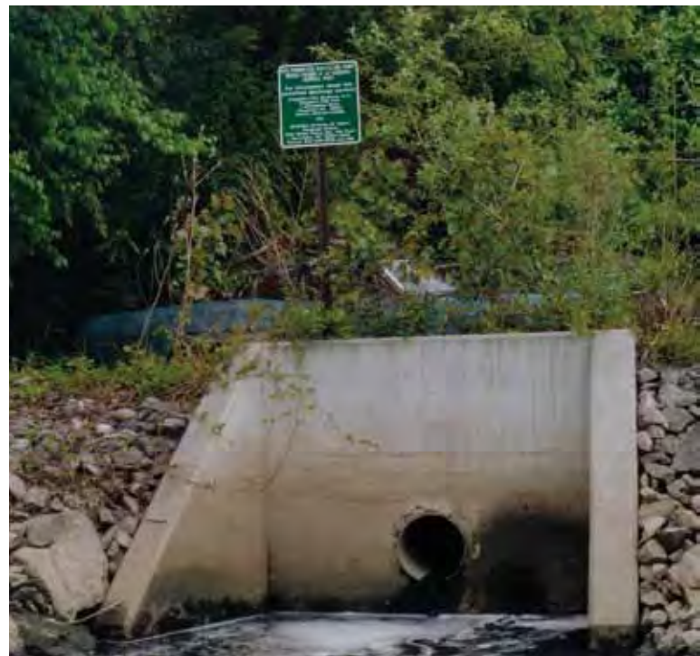
This CSO outfall discharges raw sewage and stormwater into the lower Rondout Creek, a popular swimming spot in Kingston. After the Sewage Right to Know law goes into effect in 2013, the sewage treatment plant that bypasses to this outfall will have to notify the public when they discharge.
