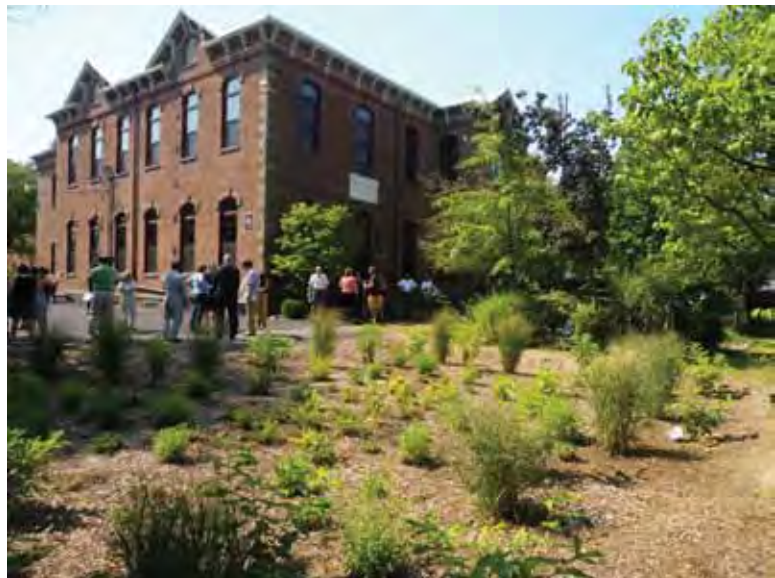
Rain Garden at the Kingston Library. The roof leaders on this building were connected to the city sanitary sewer system, carrying roof runoff to the Kingston Sewage Treatment Plant and contributing to combined sewer overflows. Now the runoff is absorbed by the rain garden.
