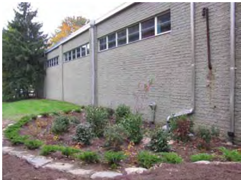
Rain Garden at the Mt. Pleasant Highway Garage. Rain gardens manage and treat stormwater by filtering runoff through soil and vegetation within a shallow depression.
