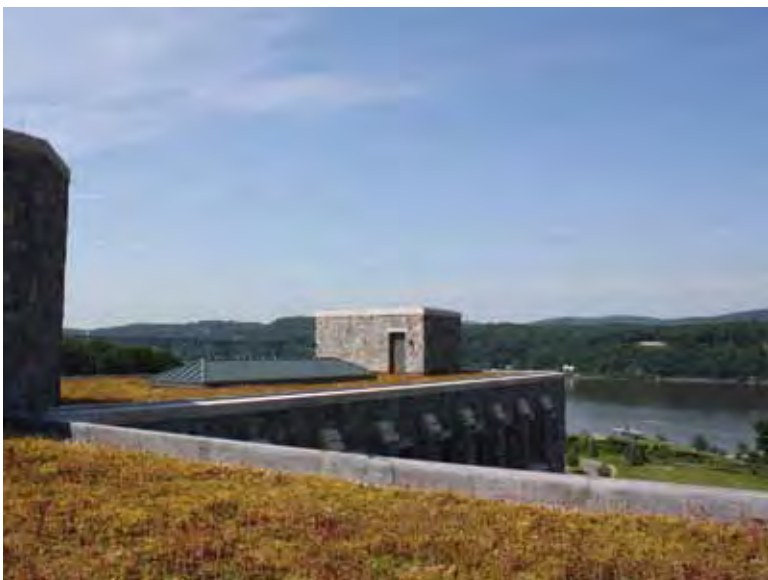
Green Roof at Marist College. Green roofs are layers of soil and vegetation installed on rooftops that capture runoff. They absorb rainwater, provide insulation and help lower urban air temperatures.
