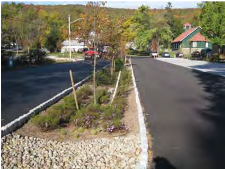
Vegetated Swale in the Village of Greenwood Lake. Swales are natural drainage paths or vegetated channels used to transport water instead of storm sewers or concrete channels. They allow for the filtering of pollutants and infiltration of runoff into groundwater.
