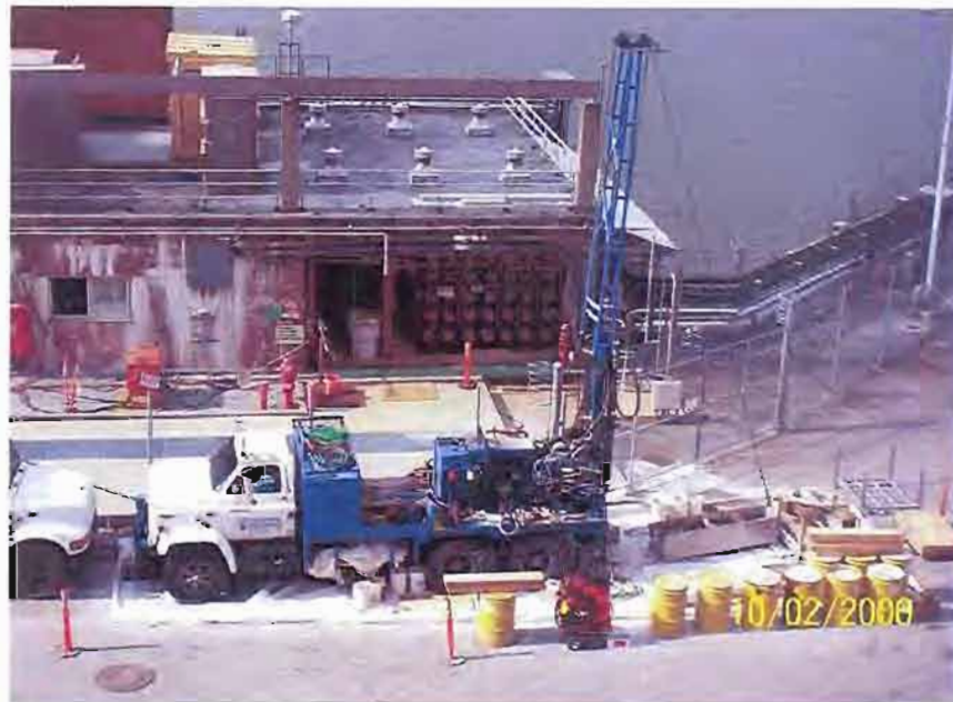
ADVANCEMENT OF BORINGS ALONG RIVERFRONT
