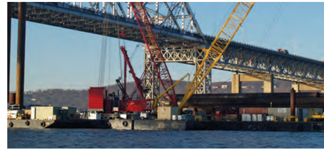
28 Protecting the River From the Impacts of Construction
