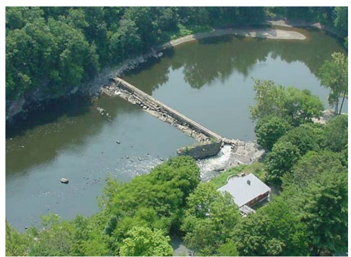
Dams create barriers to fish migration, including river herring and American eel. They also fragment habitats for resident species, degrade water quality and interrupt downstream sediment transport.
