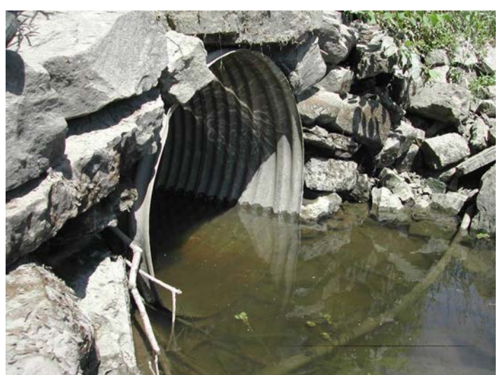
Culverts are used to pass streams and tributaries under roads or other developed properties. If not properly designed and installed, they can disrupt fish and wildlife movement and wash out during floods. (Photo: Carl Alderson, NOAA)
