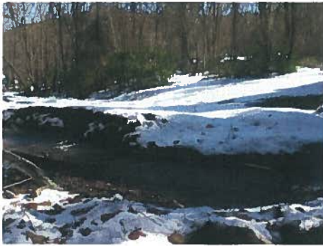
Figure 4. Area just upstream of the large dam.
