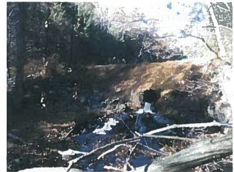
Figure 6. Dam at the beginning of segment 5.
