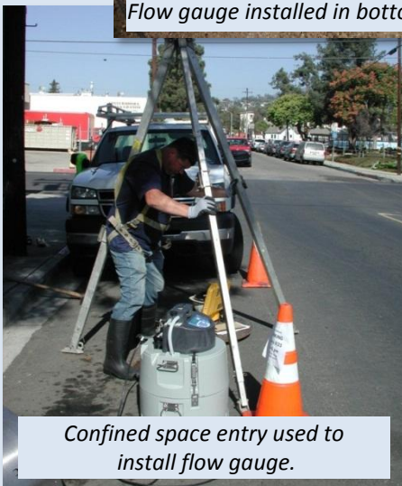
Flow gauge installed in bottom of storm drain.
