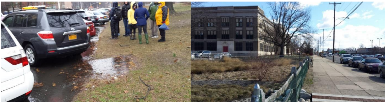
Left: runoff pooling on edge of Dickinson Avenue. Right: street runoff channeled to rain garden in Philadelphia. Photos by Korin Tangtrakul.
