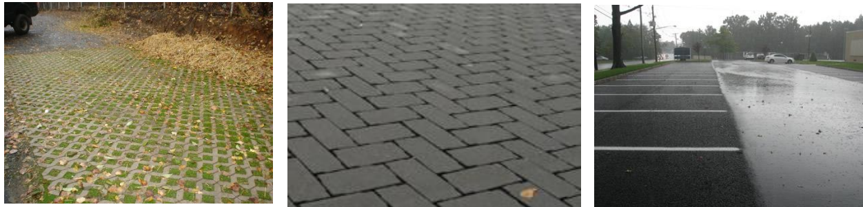
Grass pavers, permeable pavers and porous asphalt. Photos from Rutgers University.
