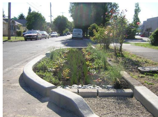
Example of a Stormwater Bumpout. Photo from Kentucky Waterways Alliance.
