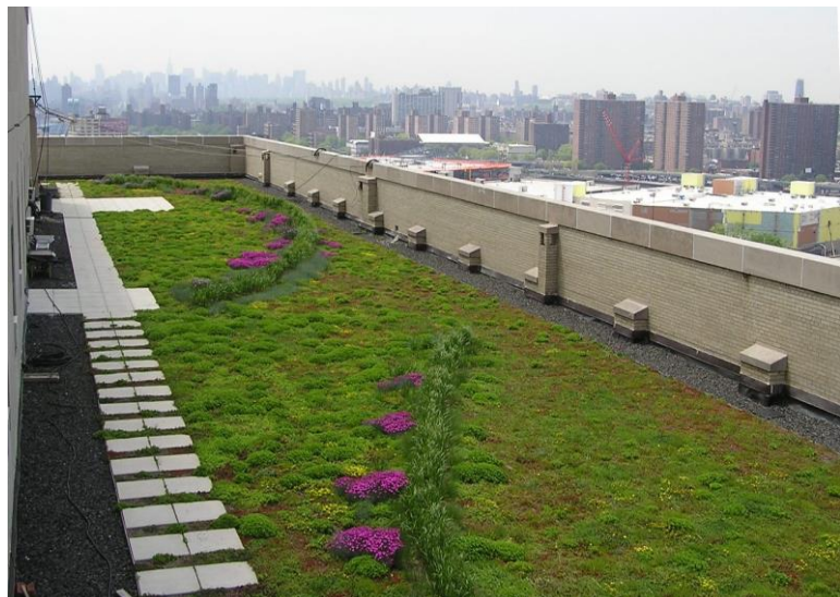
Bronx County Courthouse Green Roof. Photo from Bronx Council for Environmental Quality.
