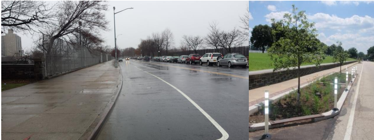
Example of a stormwater bumpout from the Philadelphia Water Department, and existing conditions along Goulden Avenue.
