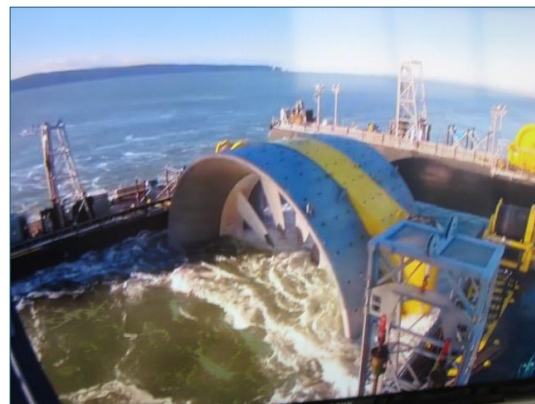
Turbine being lowered into the Bay of Fundy, where it is anchored to the bottom to capture tidal flows for power generation.
