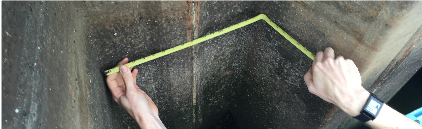
The corrugated shape of the bulkhead offers up a unique space to create habitat without interfering with functionality of the hard edge.
