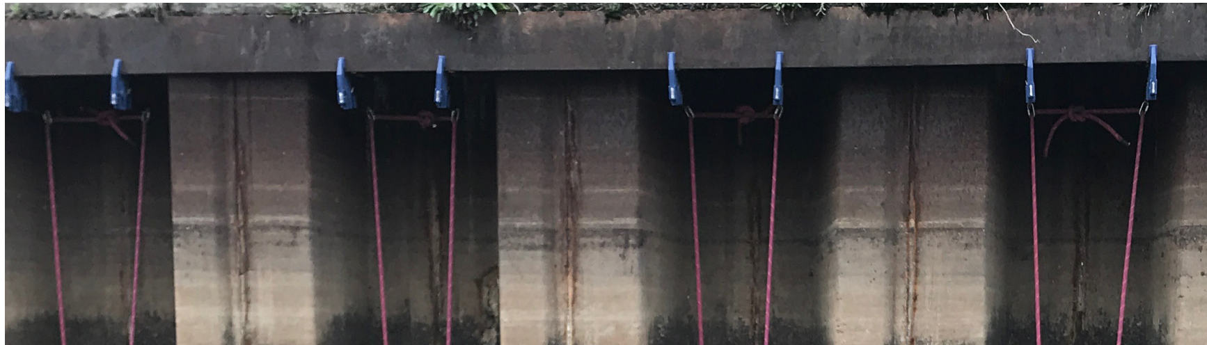
Tension rods, doubled up and used with rope, best met the project goals.
