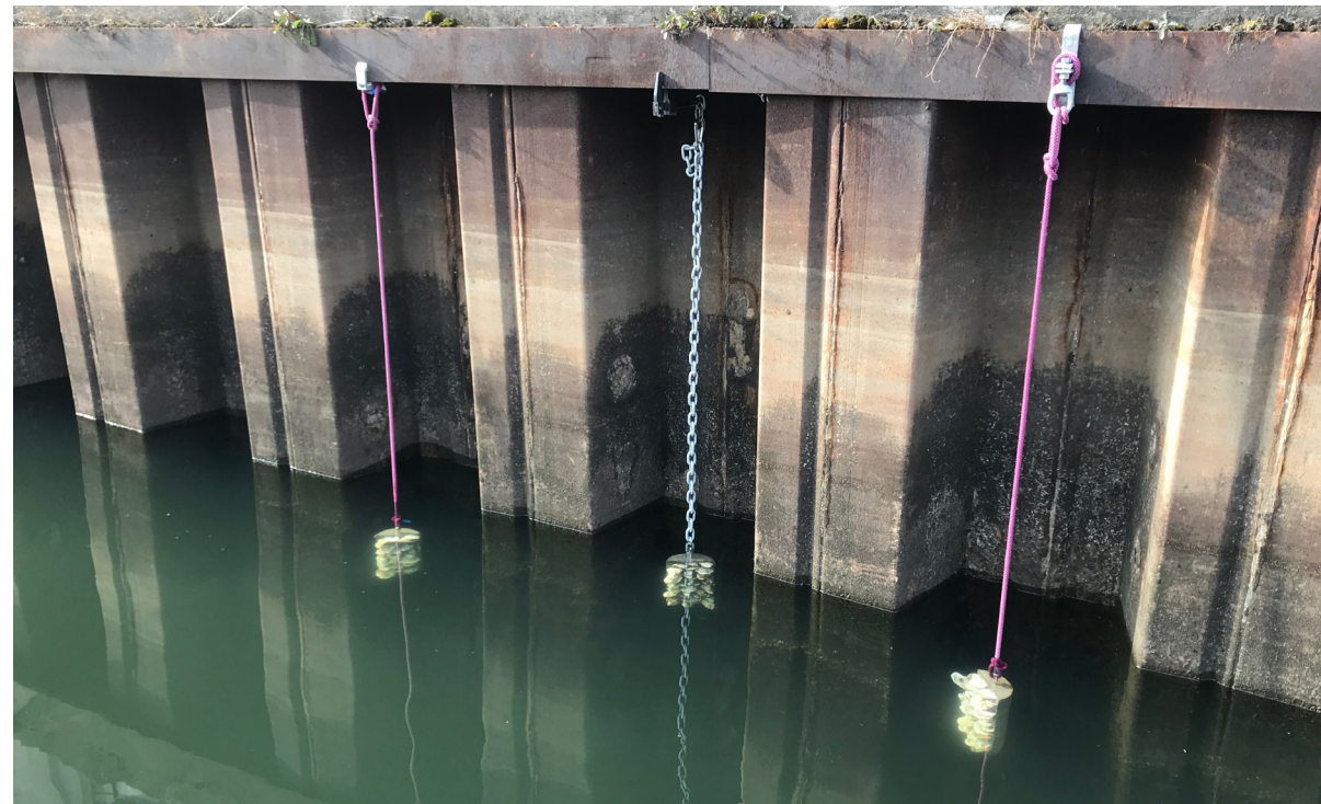
The test installation in Dutch Kills with three attachment methods.
