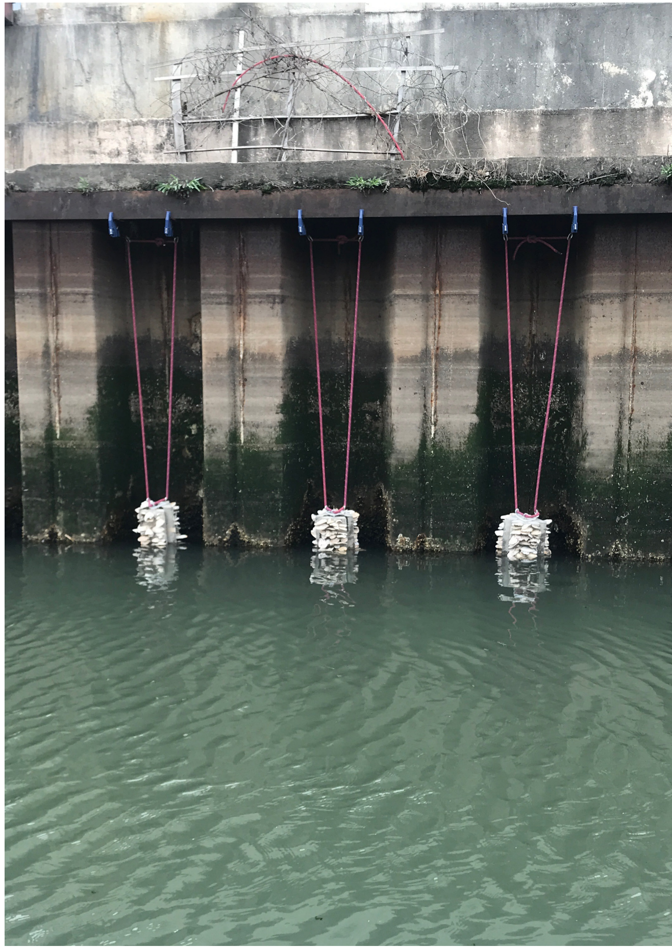
A section of the final installation in Dutch Kills.
