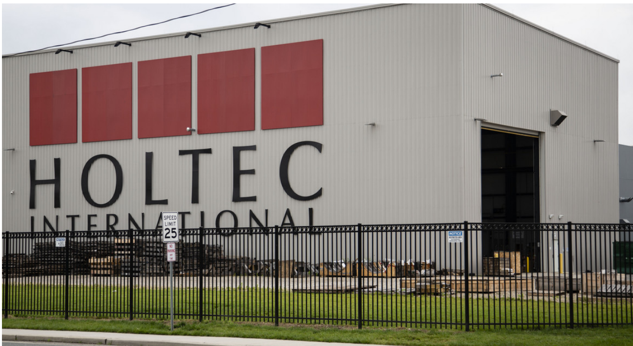
Holtec's tax credits, awarded to support construction of a new facility in Camden, were frozen by the EDA in June following a report this year by WNYC and ProPublica. | AP Photo/Matt Rourke
