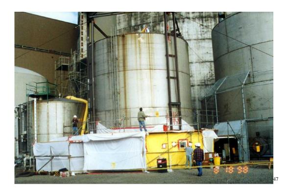
• Cutting potentially (and actually) radioactively contaminated piping at the Big Rock Point nuclear plant also used temporary ventilation modules with air flow ranges between 3,000 and 3,600 cubic feet per minute. The modules had pre-filters and HEPA filters.<sup>48</sup>
