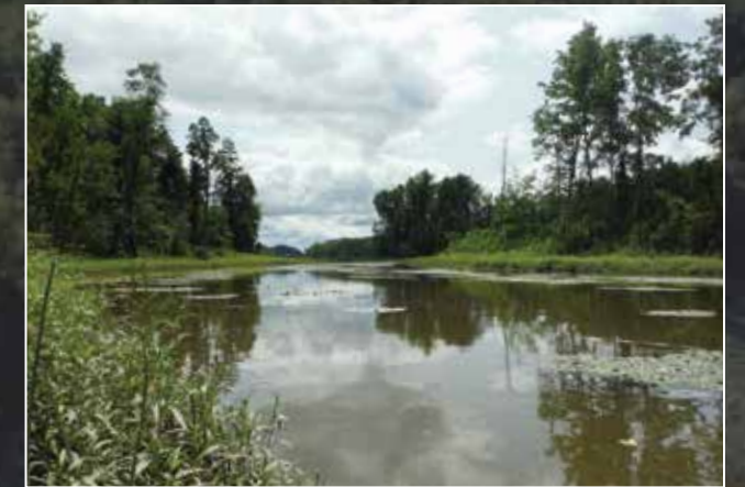
An aerial photo shows work underway in 2017 to excavate a channel at Gay’s Point in Stockport, connecting the artificial embayment at left with the main stem of the Hudson at right, and restore high quality, shallow water habitat for fish and other wildlife. The inset photo shows the newly completed channel in 2018.
