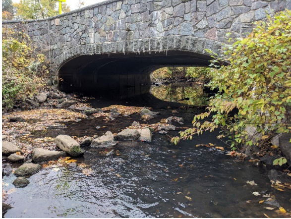
FACING UPSTREAM, OCTOBER 22, 2020
