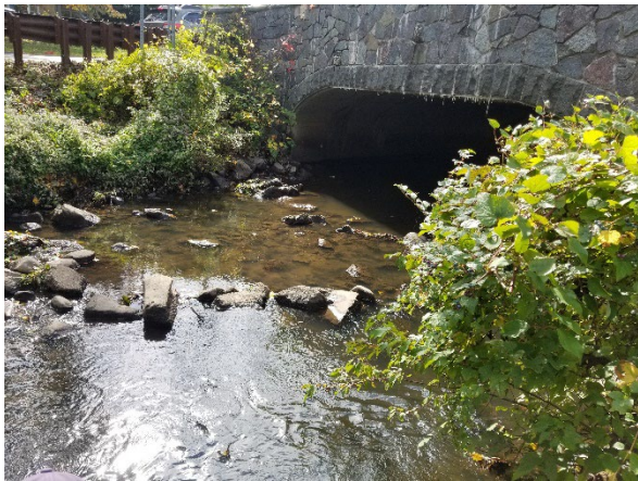
FACING UPSTREAM, OCTOBER 1, 2020
