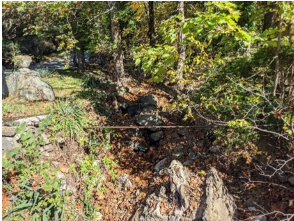
FACING UPSTREAM, AFTER TROPICAL STORM IDA, OCTOBER 20, 2021
