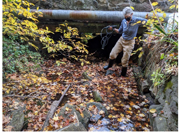
FACING DOWNSTREAM, OCTOBER 22, 2020
