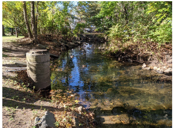
FACING DOWNSTREAM, OCTOBER 20, 2021
