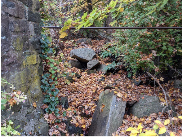
FACING UPSTREAM, OCTOBER 22, 2020
