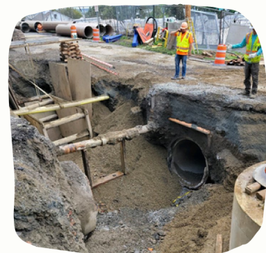
Construction on Newburgh's sewer diversion project utilizing state and federal funds.
